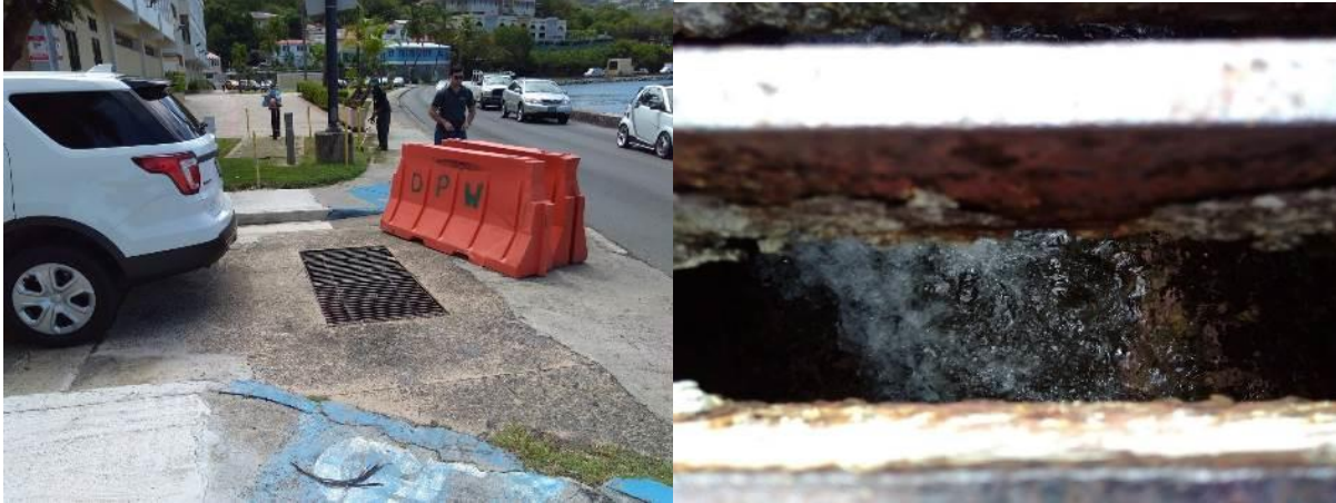
Figure 4.31: During high tide events, seawater can impede proper drainage of urban centers. Stormwater drain in Charlotte Amalie (left); closeup of wave travelling upstream in drain at low tide (right).
